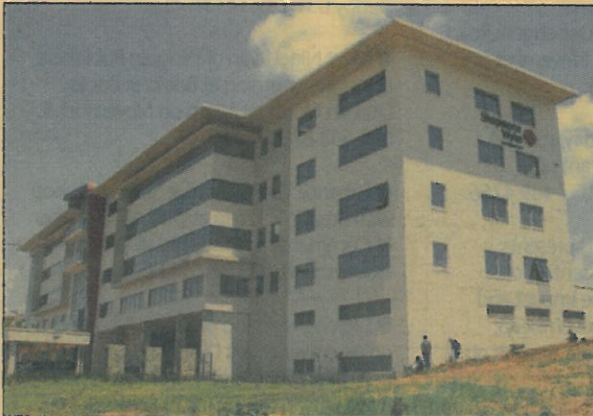
The 24 Richefond Circle Building in Umhlanga, which is home to Shepstone & Wylie Attorneys, is the first building in Durban to get both the 4 Star Green Star SA – Office Design v1 and 4 Star Green Star SA – Office As-Built v1 rating by the Green Building Council of SA. PICTURE: JACQUES NAUDE
