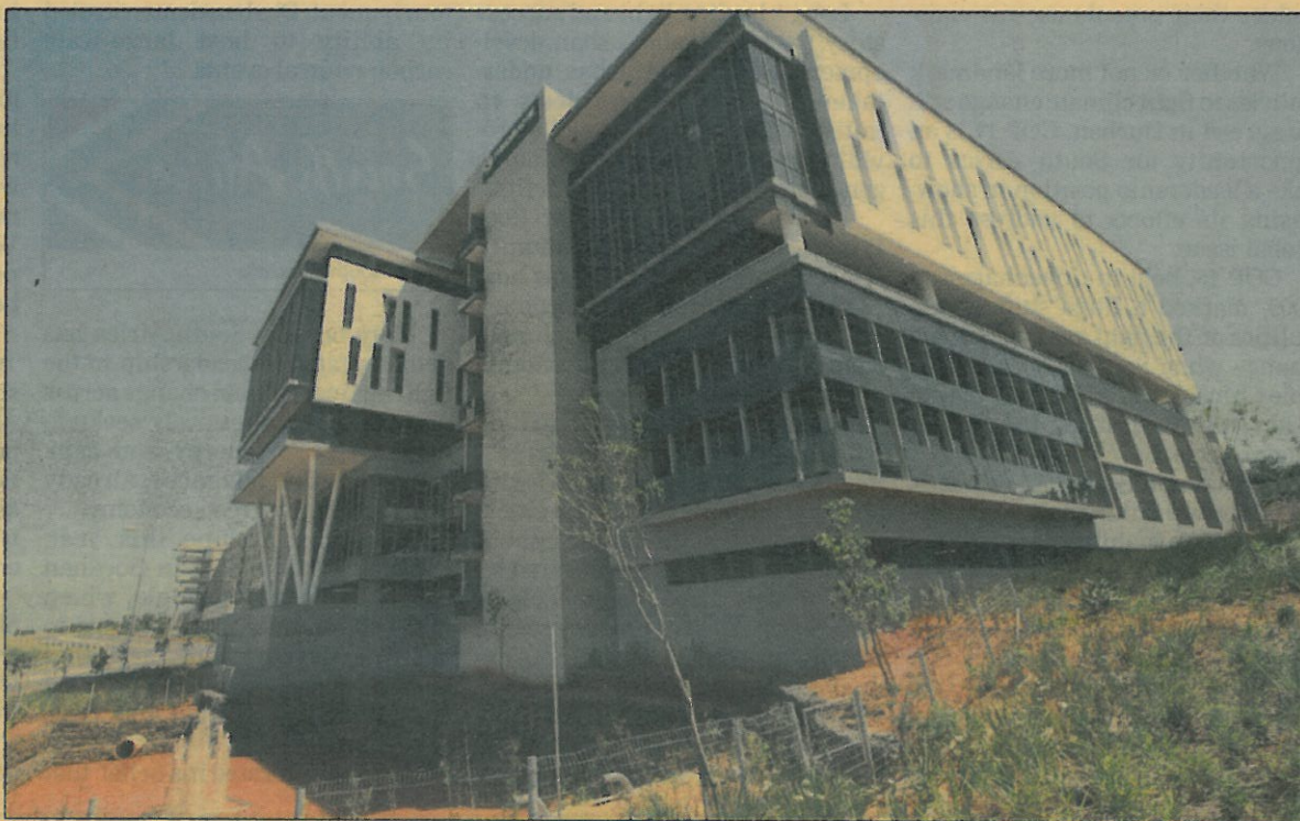
The Nedbank Ridgeside Office Development in Umhlanga, which boasts a 4 Star Green Star SA – Office Design v1 rating from the Green Building Council of SA. PICTURE: PETER HASSALL
