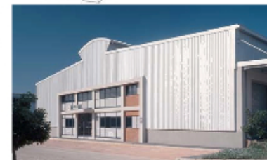
Characteristic of this development, the ridge is capped with a continuous monitor and the entrances are framed.
